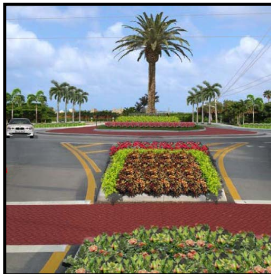
The new roundabout at Saddle Club Road & Lakeview Drive is complete.
