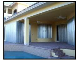
changes when windows or doors fail. Shutters can be made of metal, wood or plastic and are available in different styles; the most common are steel or metal panels, accordion style and roll-down.
