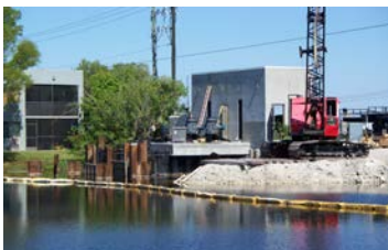
Pump Station Upgrades and other Water and Sewer System Improvements
