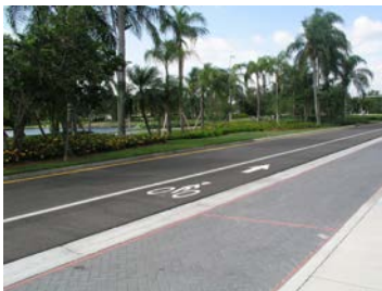
Bike Lane Upgrades
