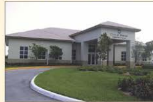
Community Center & City Park Improvements
