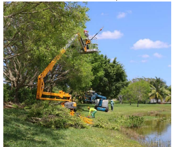
Tree Trimming of Back Berms Along South Post Road
