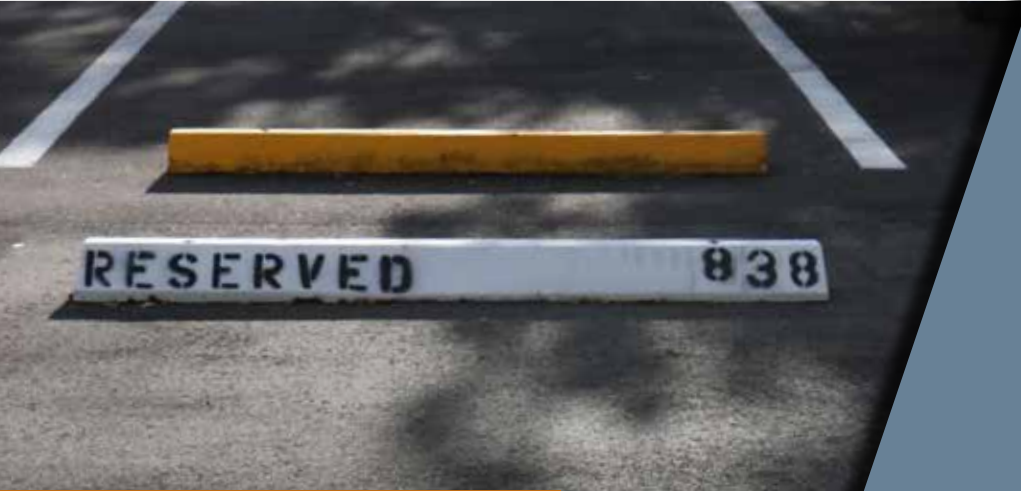
Well Maintained Wheel Stops
