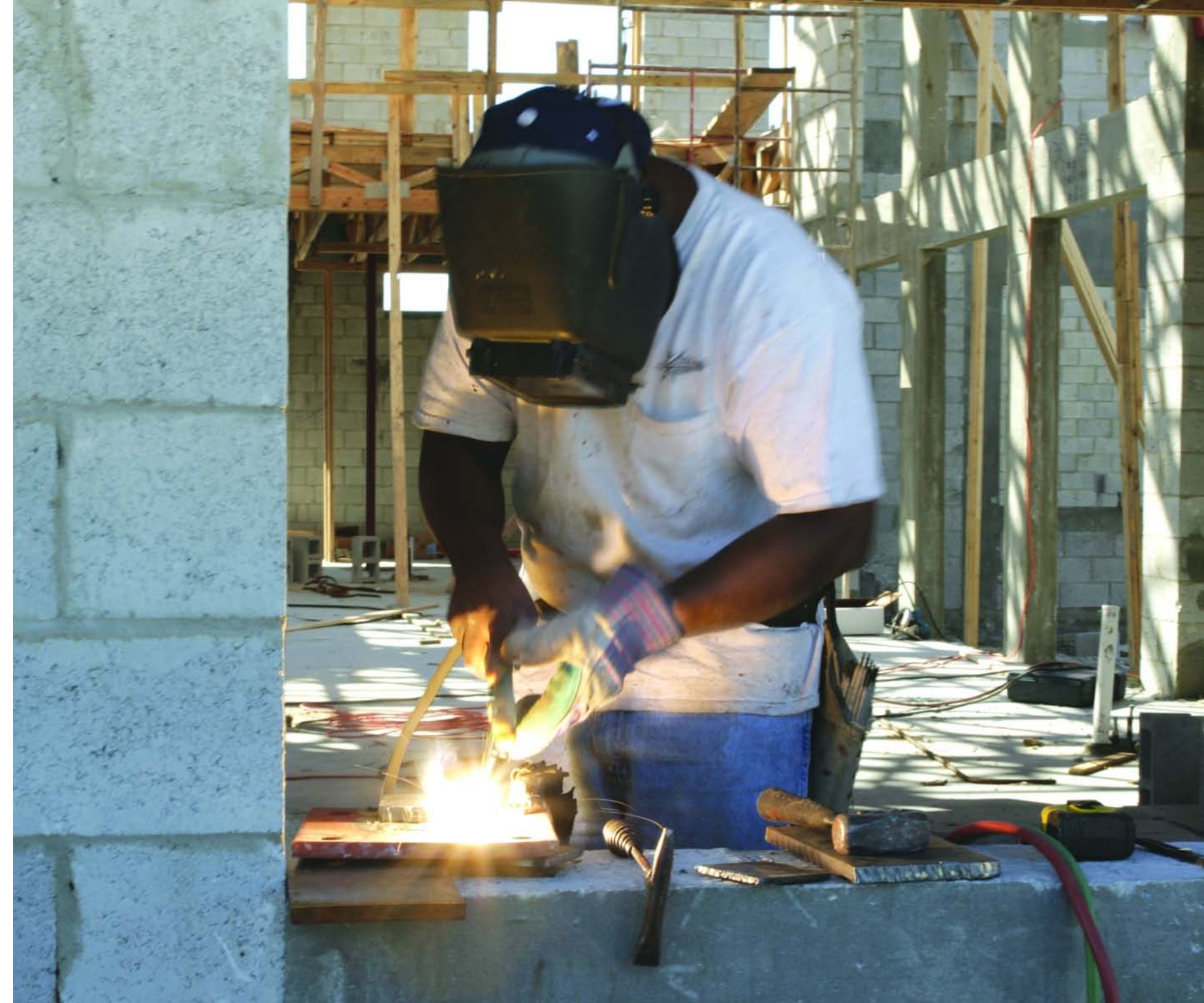
Home construction at Windmill Reserve
