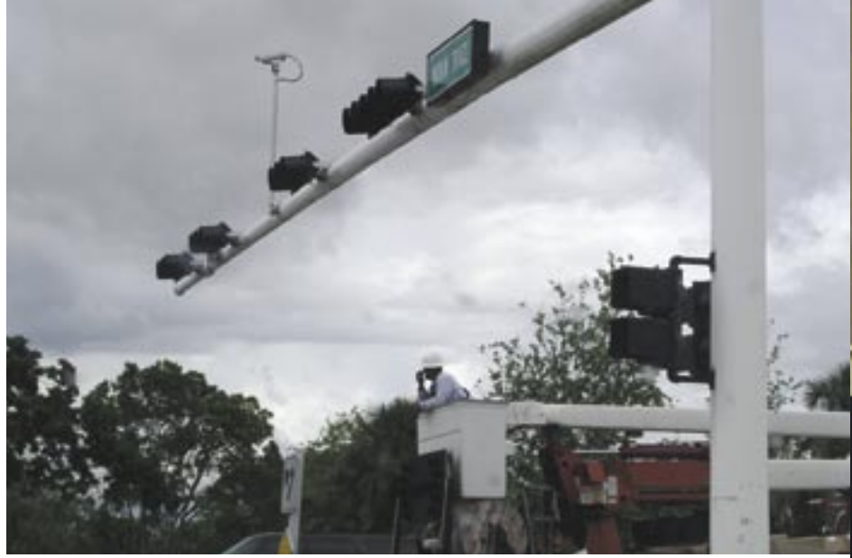
Signal heads changed to a horizontal mount at all Weston intersections.
