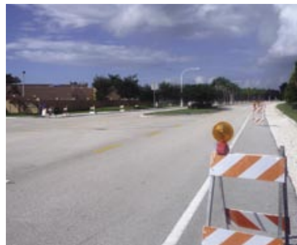
West Side of Manatee Isles Drive prepped for new curbing
