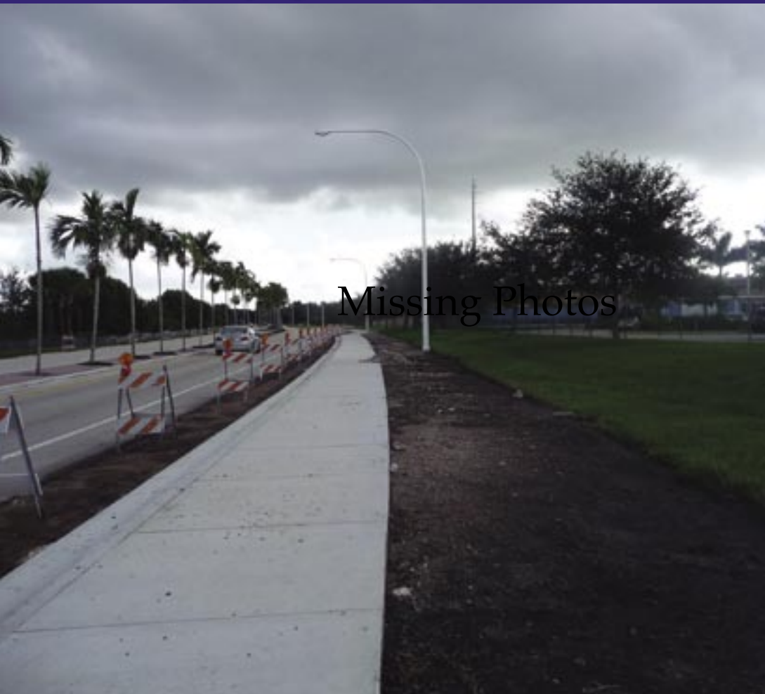
Newly installed curbing and gutters adjacent to Manatee Bay Elementary School
