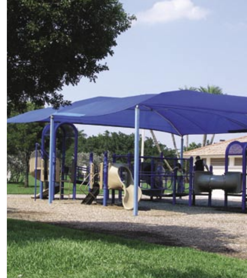
Library Park Construction
