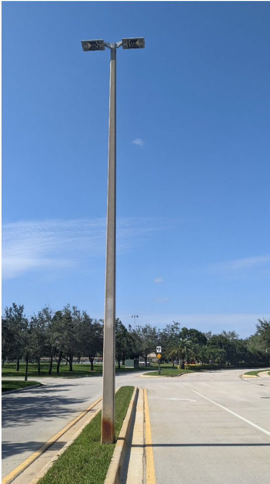
Concrete Light Poles (City Facilities - Parking Lots)
