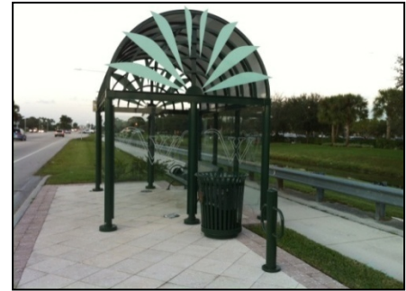
Bus Stop Shelters on Weston
